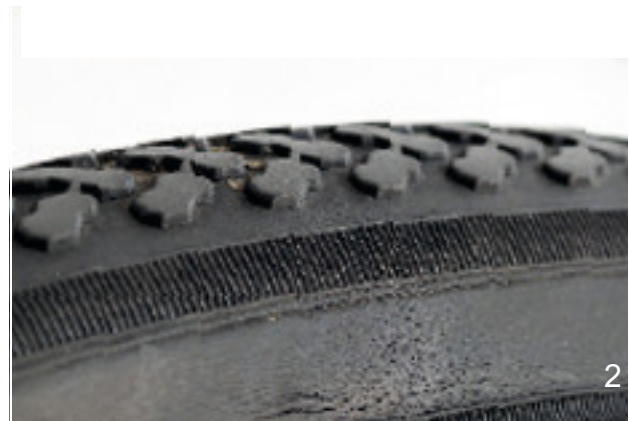
Figure 149: Examples of fatigue cracks (1) and ageing cracks (2)
